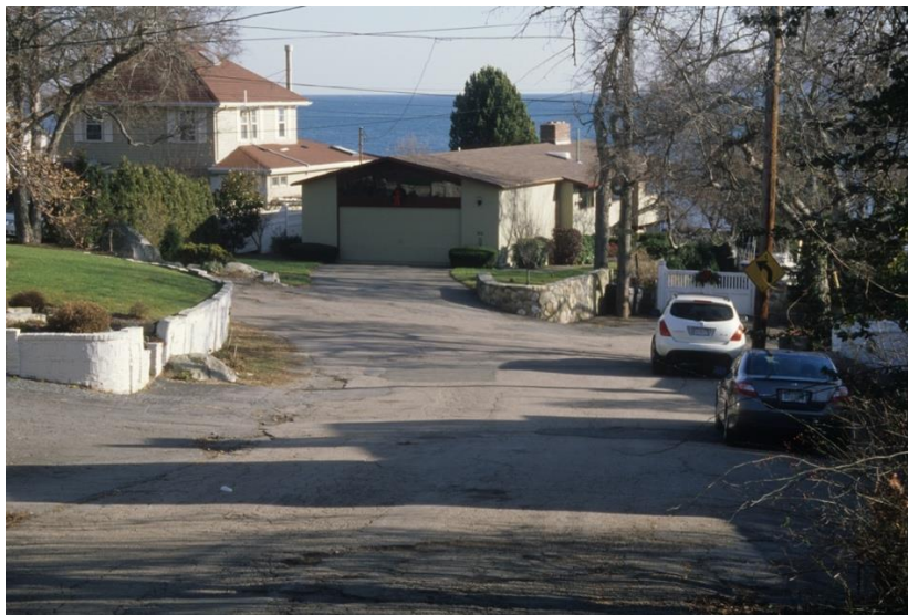
FIGURE 4 A VEHICLE DROVE INTO THE HOUSE LOCATED OUTSIDE A CURVED ROAD AROUND MIDNIGHT
